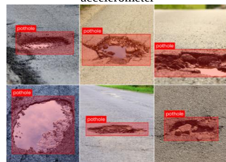
Figure 6 Identifying potholes using a camera
