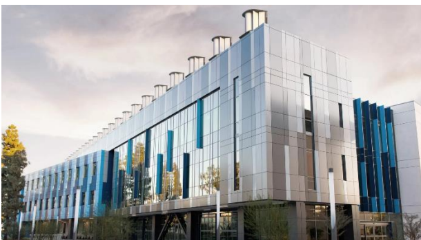
Figure 4 Installation of the Aeromine passive wind turbine system on a building [24]
