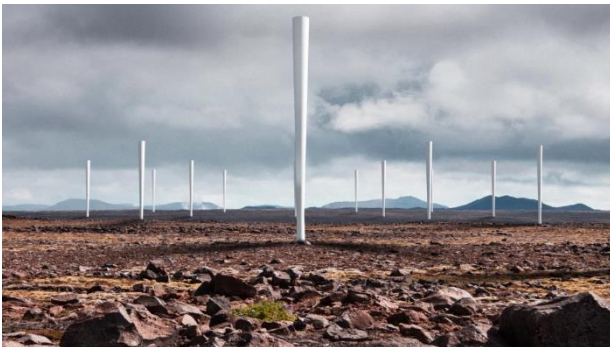
Figure 2 Wind energy system with bladeless turbines [20]
